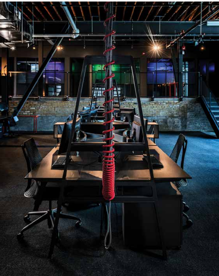
This page In response to a heritage building where limited alternations to walls and floors were allowed, Quadrangle made extensive required cabling a prime feature. Bright red auto-body shop hose coil contains the electrical and data cabling down from above.
